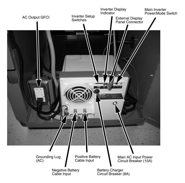
Figure 8. Power Pallet Features and Safety Devices (120V)
